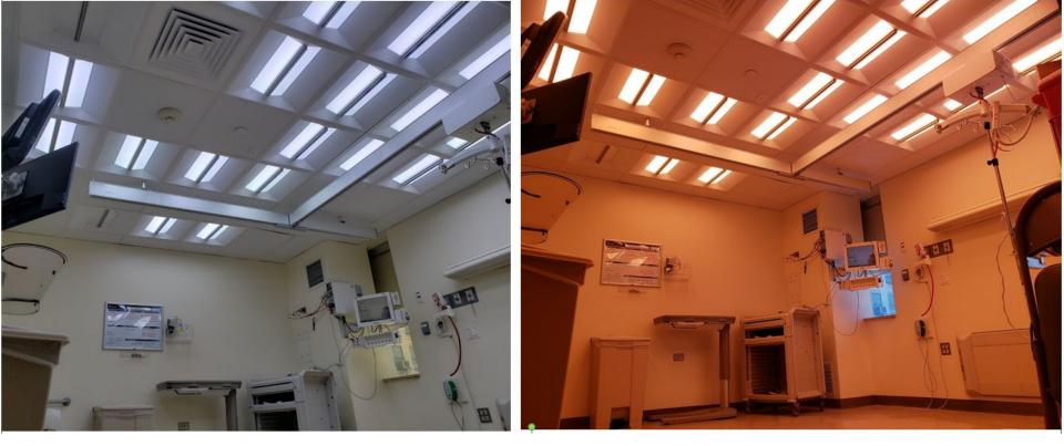
Shown above left are Telelumen Octa Light Players set to a mode enriched in short wavelengths and above right is the same system enriched in long wavelengths at an intensive care unit (ICU) in the Jefferson Hospital for Neuroscience in Philadelphia, PA (2019).
